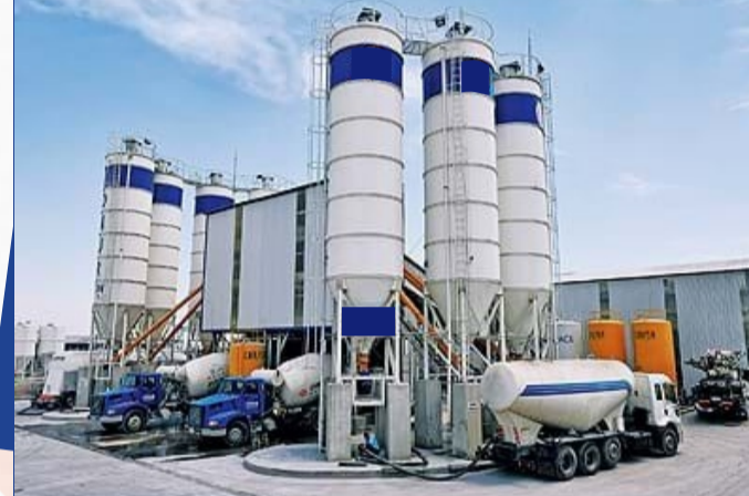
Concrete Batching Plant
